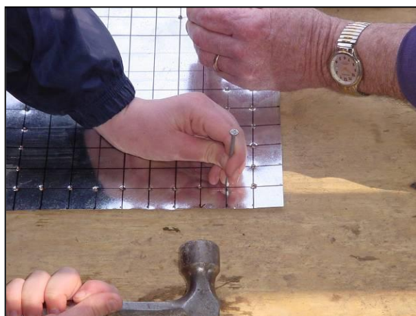
Drawing a grid will help with the nail-hole placement
